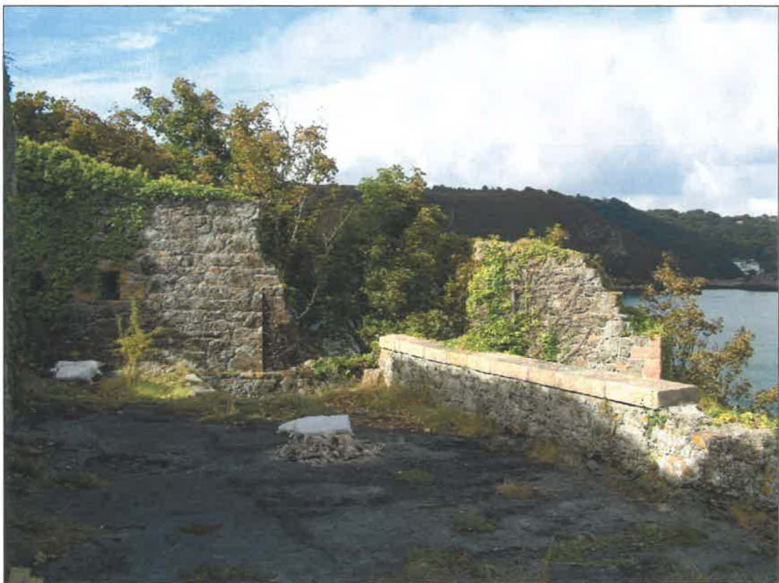
Fort entrance and platform above the guardhouse showing damage to the western flanking wall and wall tops
