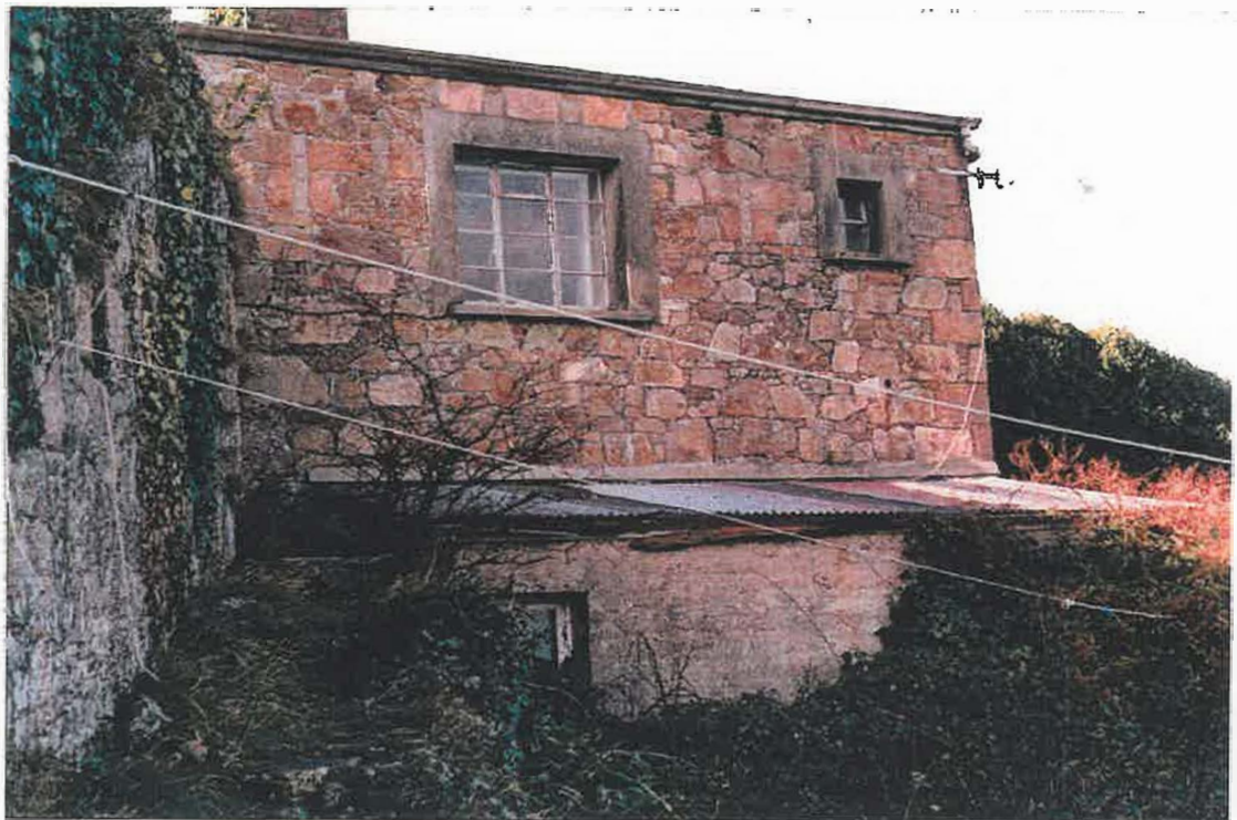
6: Lean-to structure recommended for demolition.
