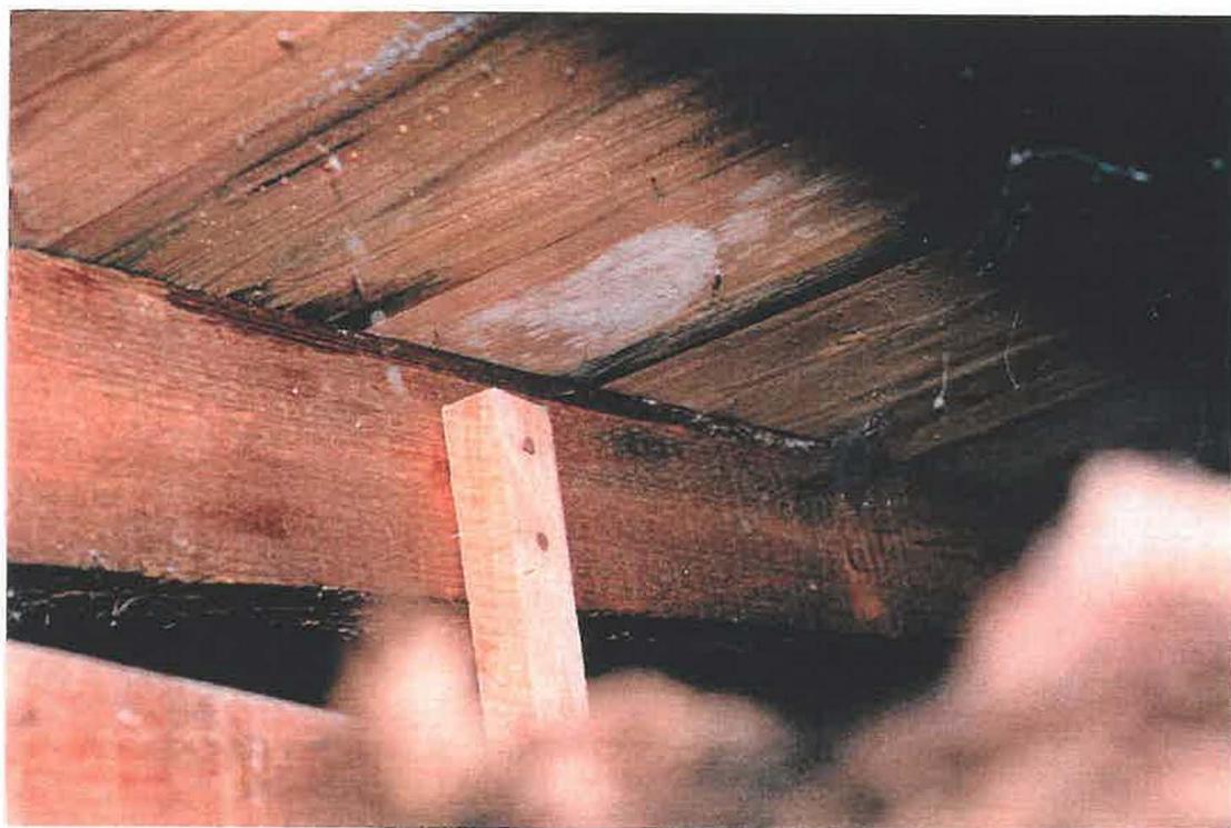
10: Guard House roof - timber decay.
