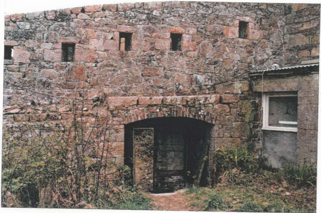
7: South battlement - Doors requiring extensive restoration. (Note also loose pavings and copings).
