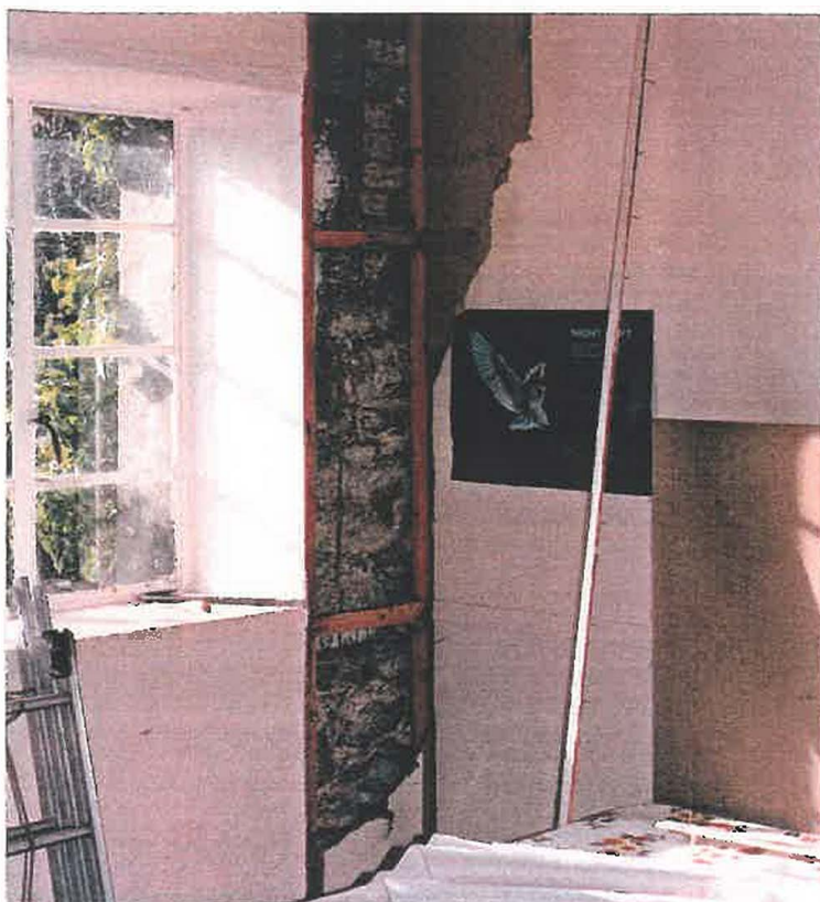
9: Guard House - First floor interior showing recent work to form window opening.
