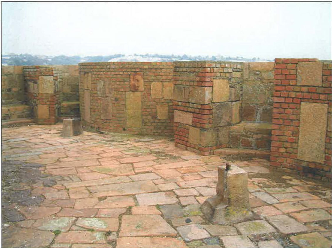
1795 traversing gun platforms with 1940s insertions
