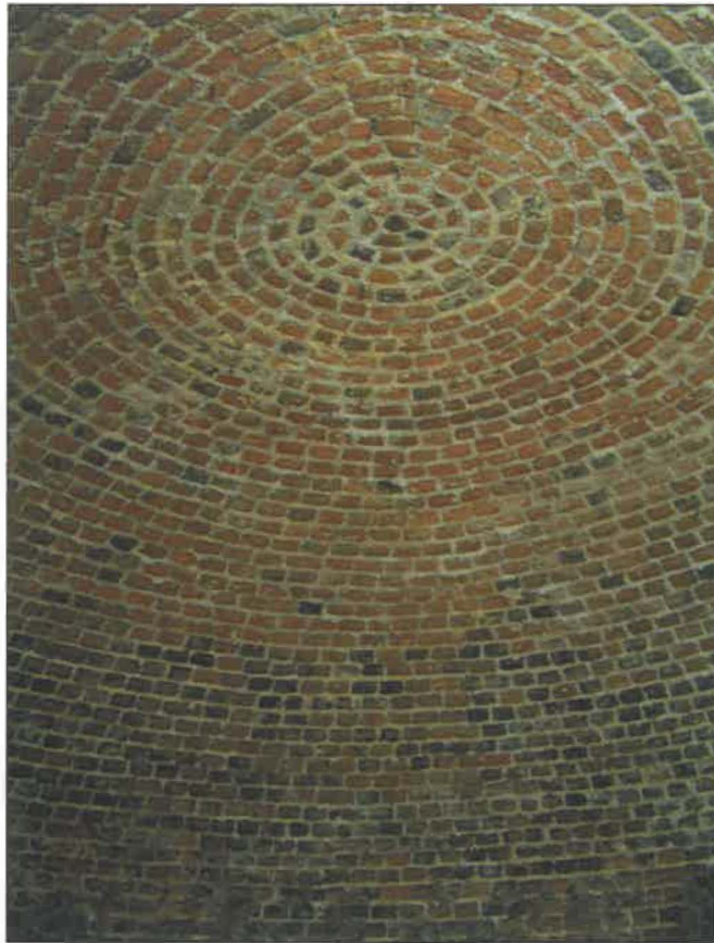
brick vaulted magazine
