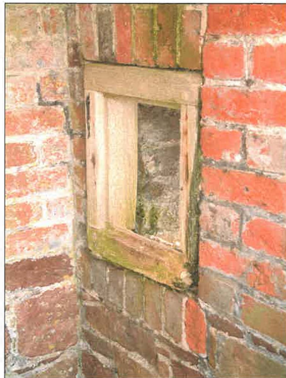
original timber framing inside machicolation
