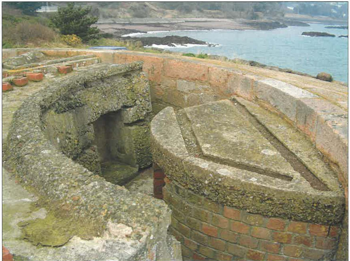
1795 traversing gun platforms with 1940s insertions
