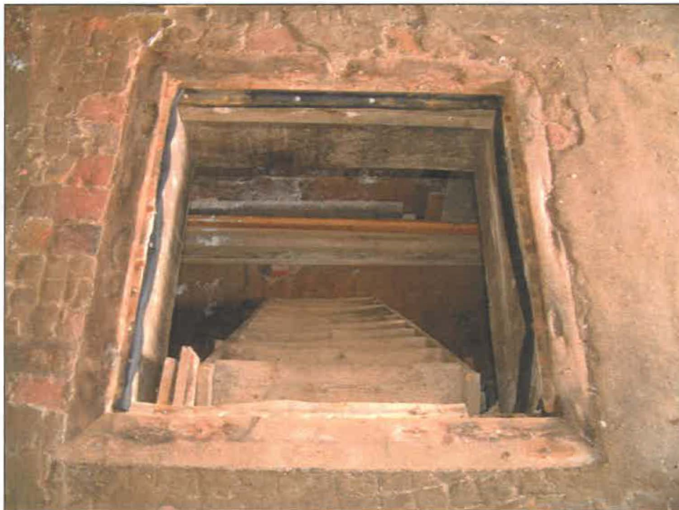
Entrance hatch to magazine on lower level (detail of German repair to hatch door)
