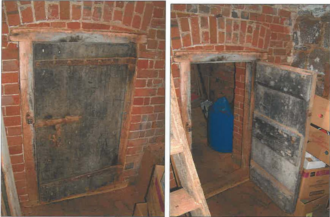
West magazine / storeroom showing original timber door and ironwork
