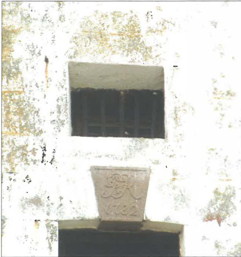
Entrance into tower showing 1782 keystone and original iron bars to window opening
