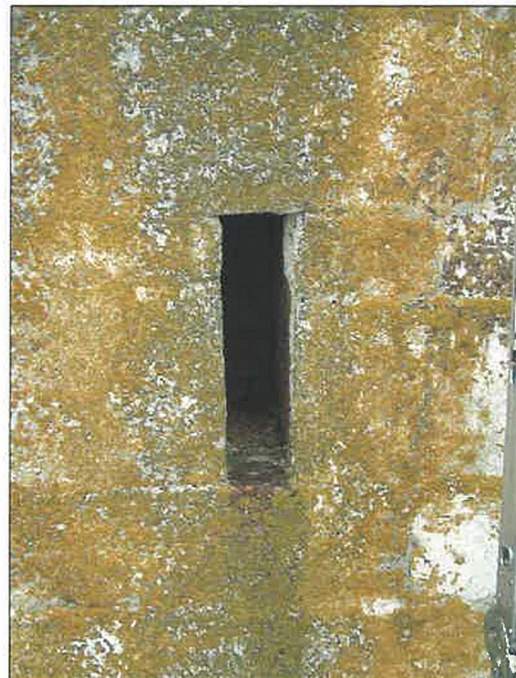
Detail of ventilation slot on interior of magazine and on exterior of tower
