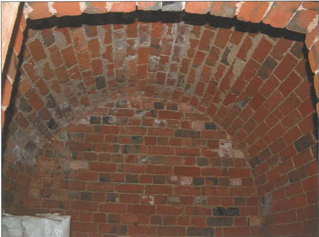
East magazine / storeroom showing brick vault
