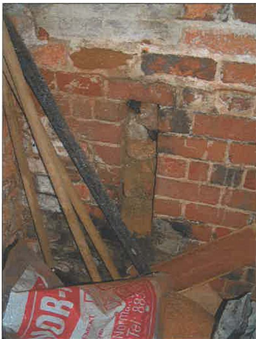
Detail of ventilation slot on interior of magazine and on exterior of tower
