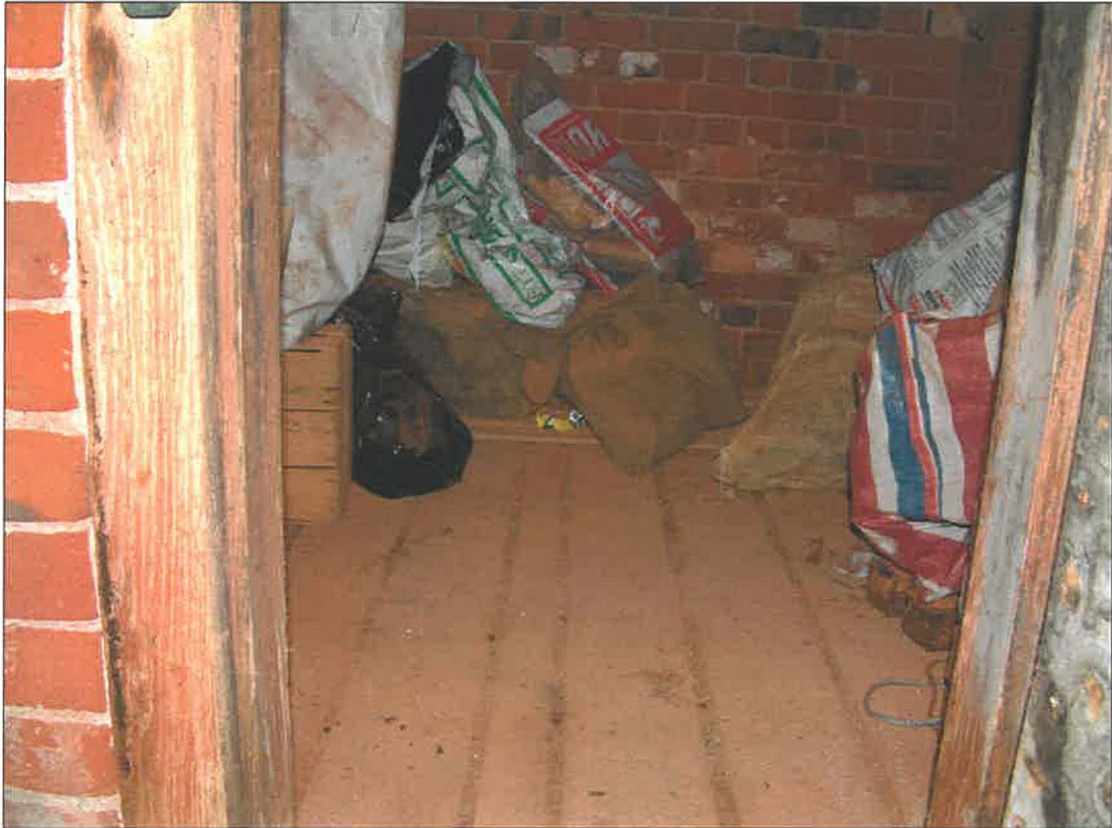
East magazine / storeroom showing softwood floor laid on sand
