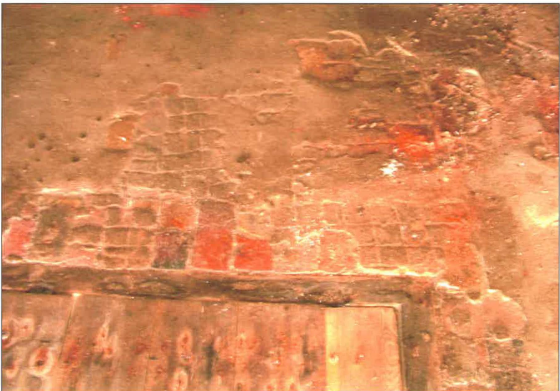
Brick floor with mortar finish (top of brick vaulted rooms below)
