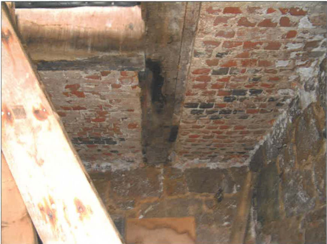
Lower level showing timber beam and underside of brick floor
