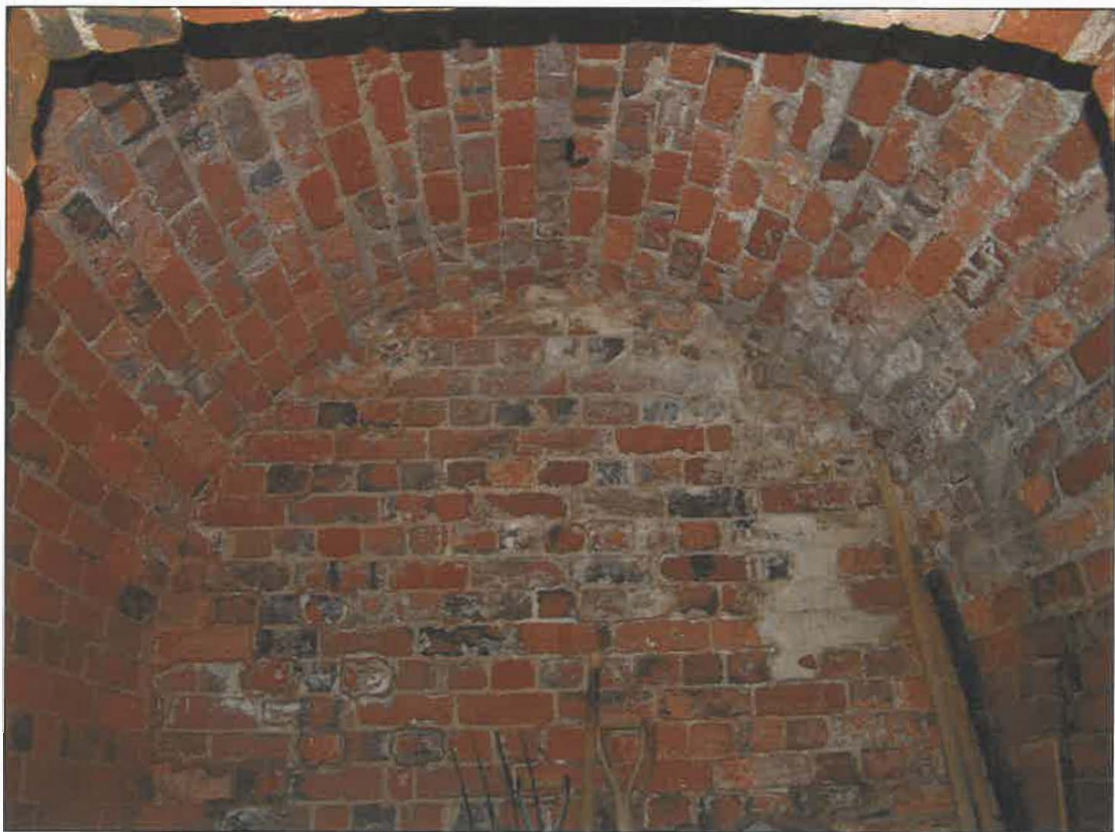
West magazine / storeroom showing brick vault
