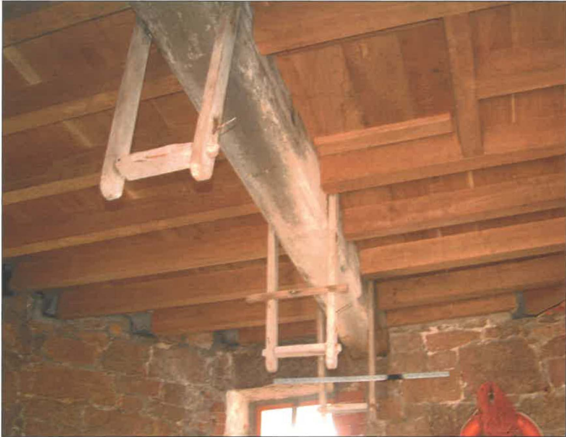
Original timber beam with storage rack and replacement timber floor to upper level
