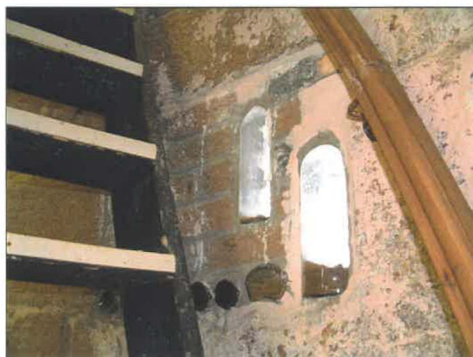
detail of window blocked with bottles and brick
