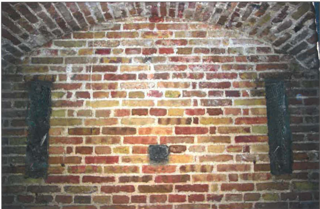
east wall of inner cell showing ventilation slots
