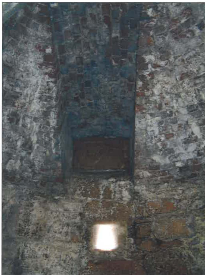
example of loophole with window above
