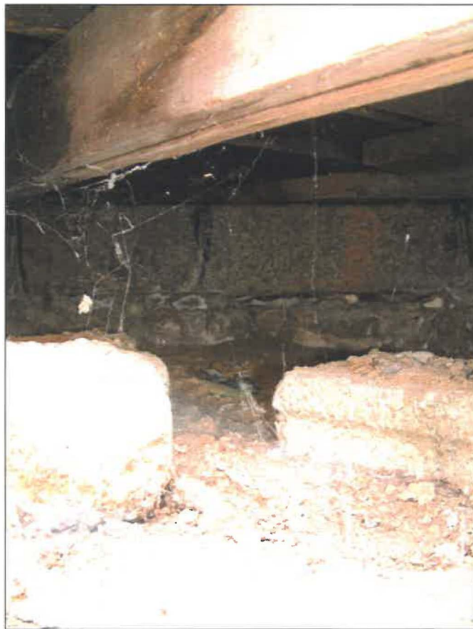
firing step now underneath modern timber decking
