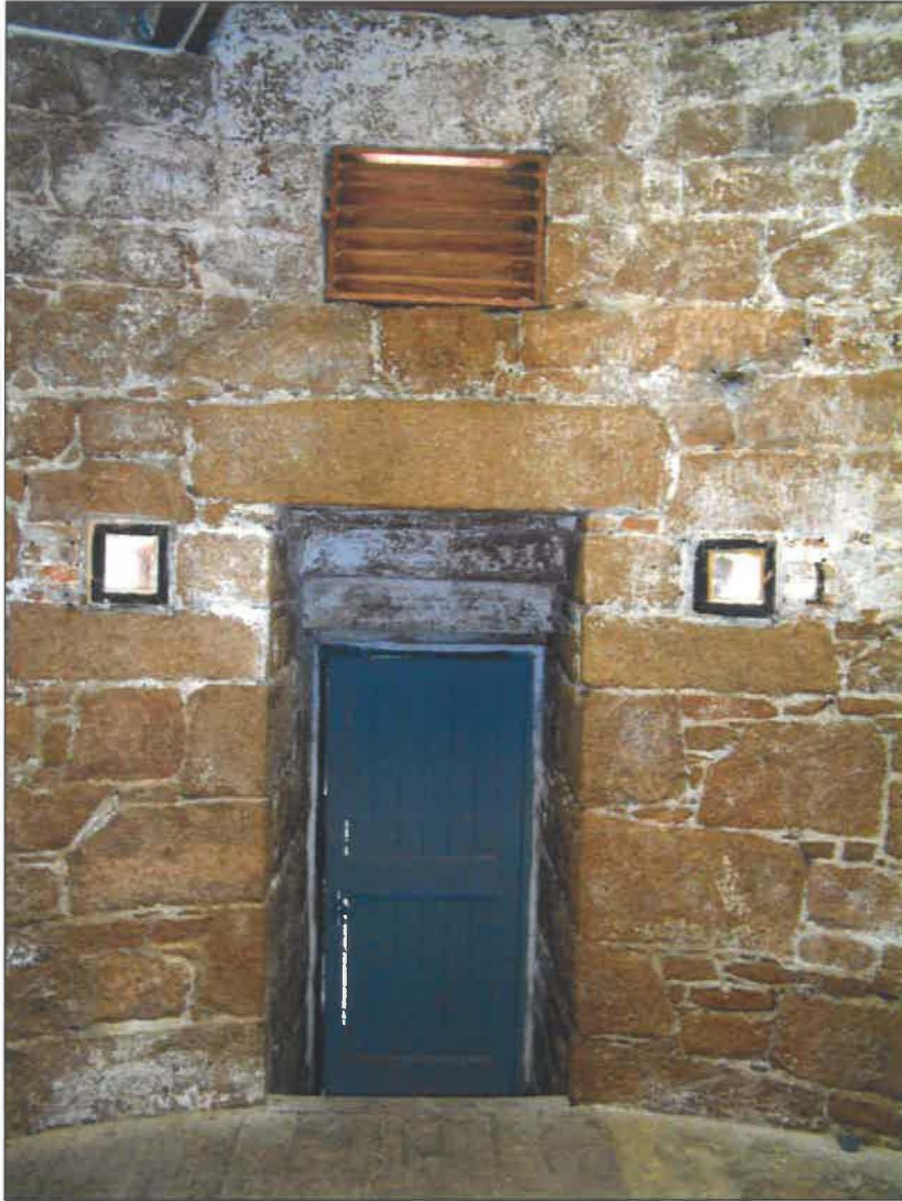
doorway with gun loopholes to each side and window above
