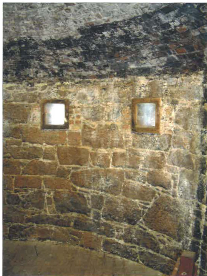
granite walls with brick vault and timber floor
