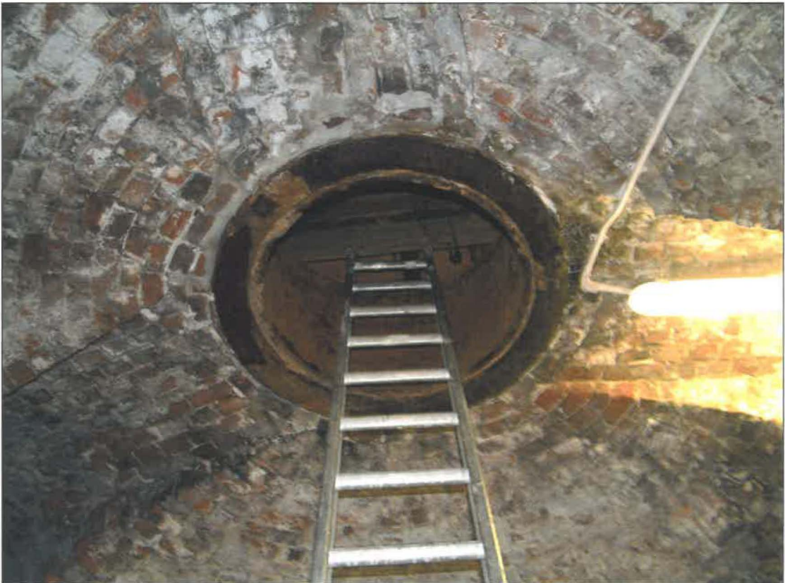
central access hatch to gun platform
