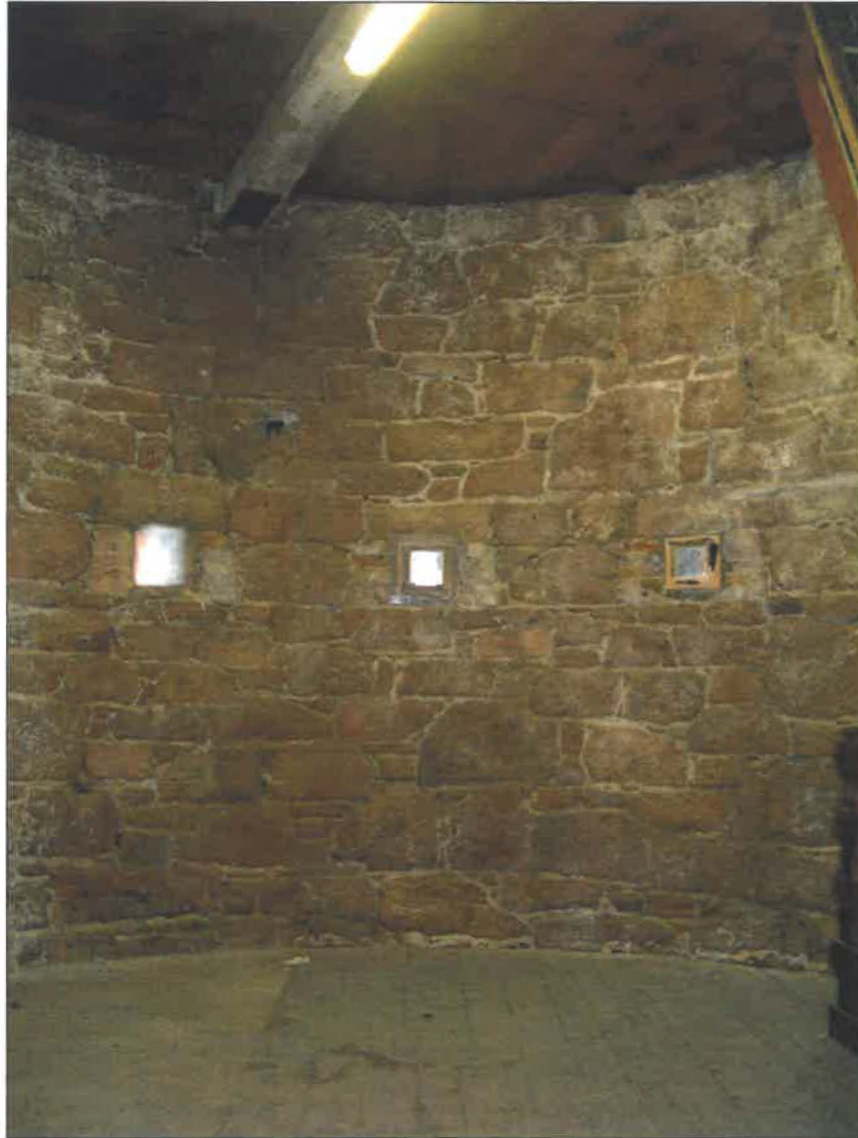
circuit of loopholes with timber beam above
