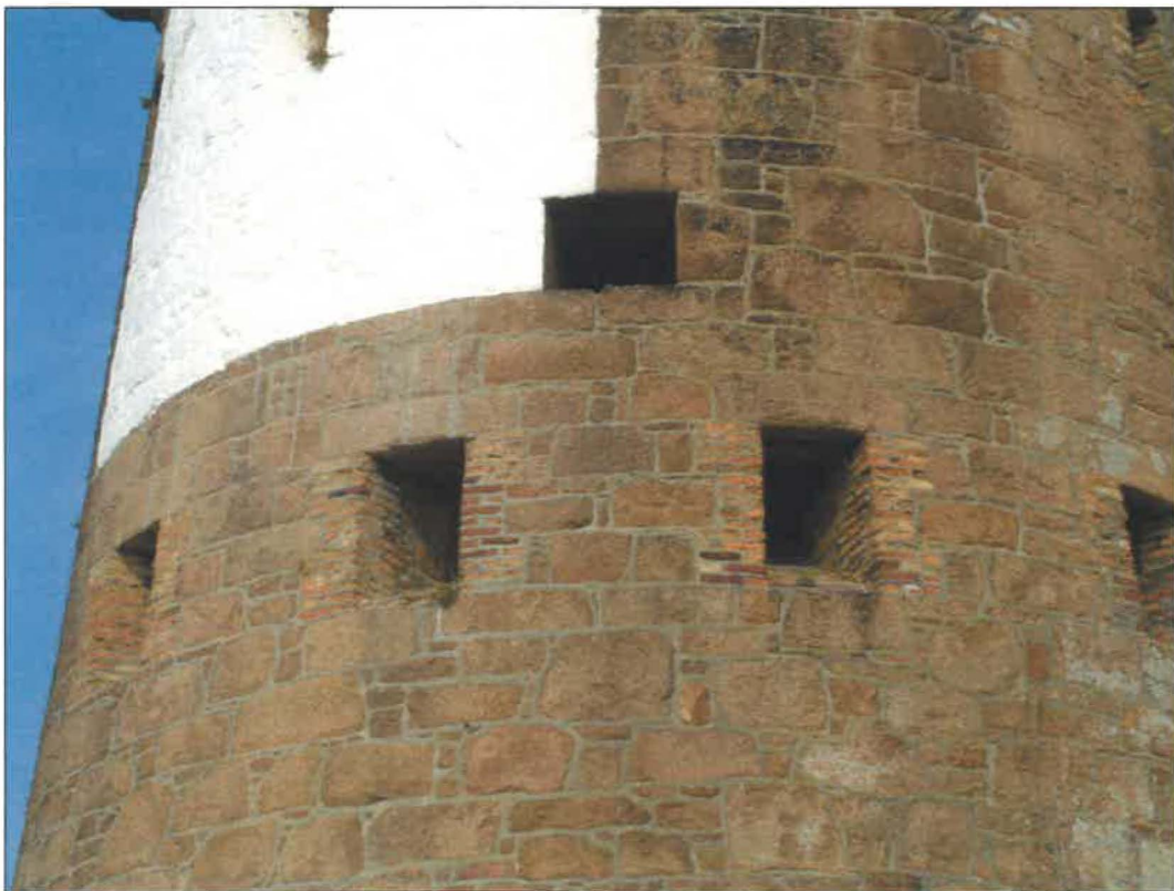
detail of doorway, gun loopholes, windows and ventilation slot
