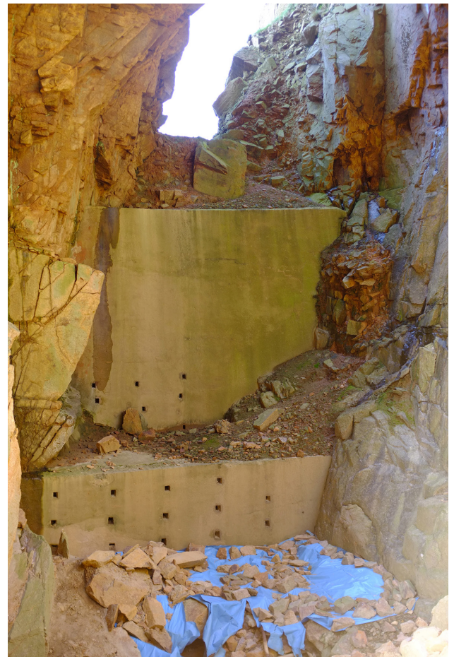
Figure 36: Partially filled 'deep sounding' below plastic sheet
