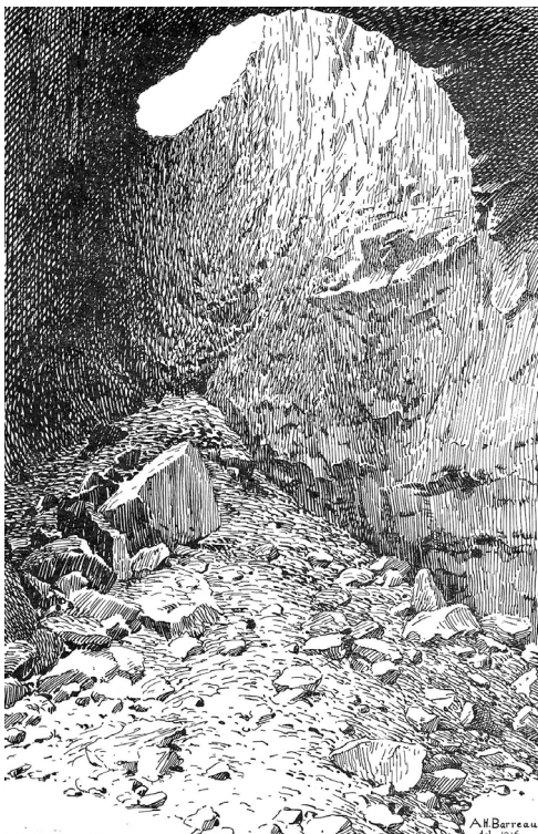
Figure 14: After the collapse of 3 September 1915
