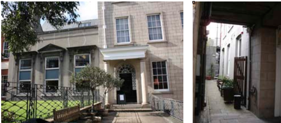
Figure 1.8 The front entrance with Billiard Room to the side, cellars below, the bays on the west side having been removed.
