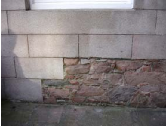
Figure 1.2 Base of north wall, possible remnants of an earlier structure
