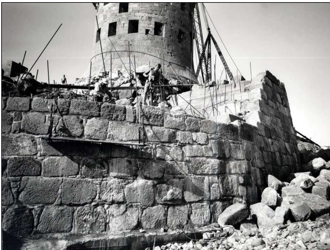
photograph of repair works underway
