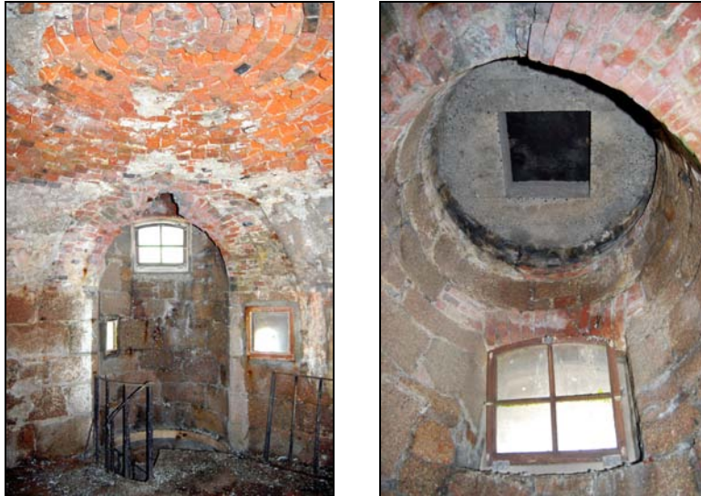
access to roof platform
