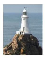
the world to be built from reinforced concrete rather than traditional stone blockwork and its light could be seen for up to 18 miles.
