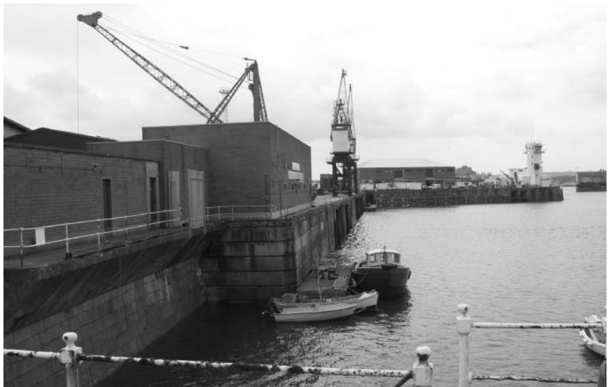
Detail of the Victoria Pier at St Helier Harbour.
