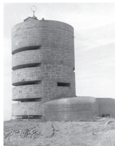
The reinforced concrete German coastal artillery tower at La Corbière was originally camouflaged to resemble an 18th-century Jersey granite round tower (Courtesy of the Société Jersiaise Photographic Archive)
