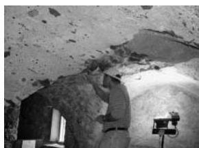
Delicate restoration work is carried out on the undercroft.
