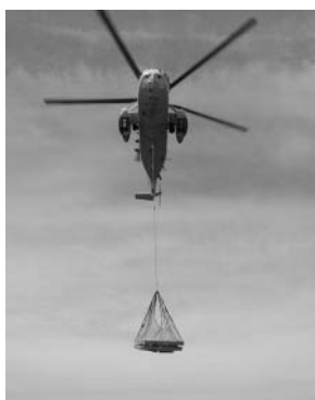
A helicopter airlifts the oak floor beams into Mont Orgueil.
