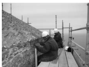
Carpenters restore the oak fascia on the North East Tower.
